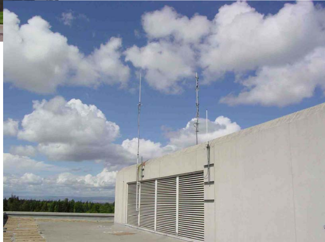
A view from the roof looking at the antenna (W6TDM antenna is on the left).
