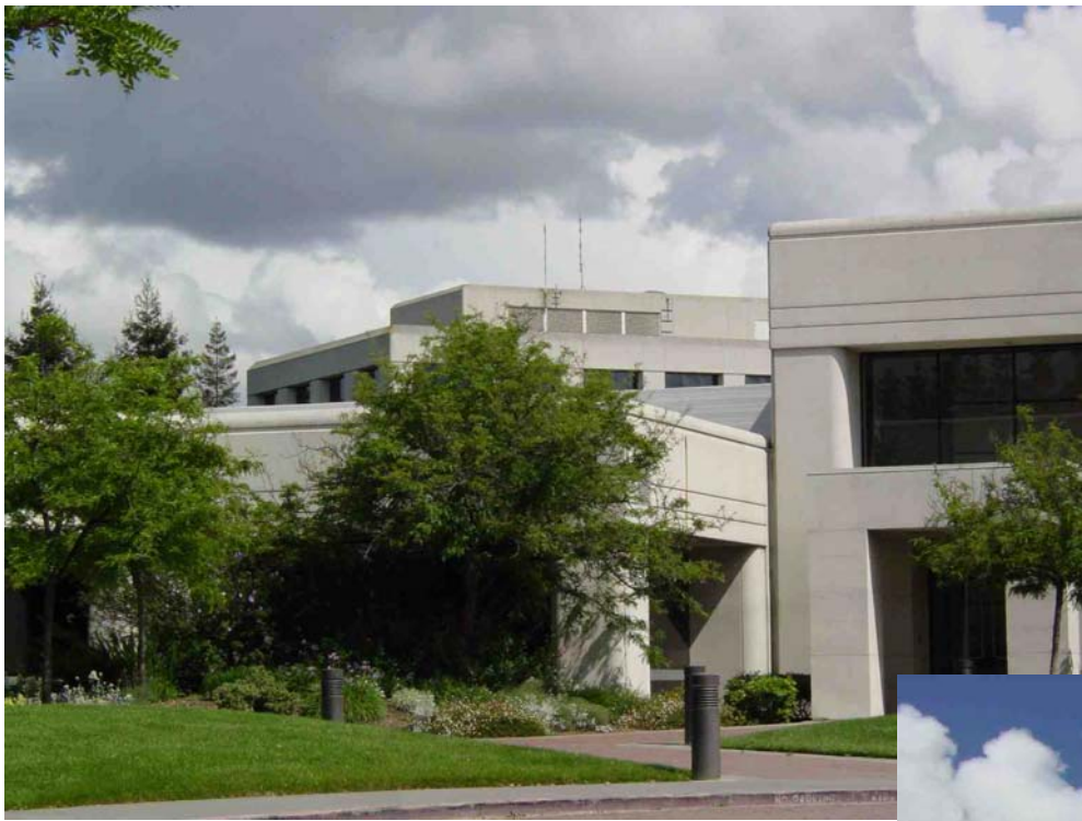
A picture taken of the repeater site near the intersection of Tantau Avenue and Vallco Parkway.
