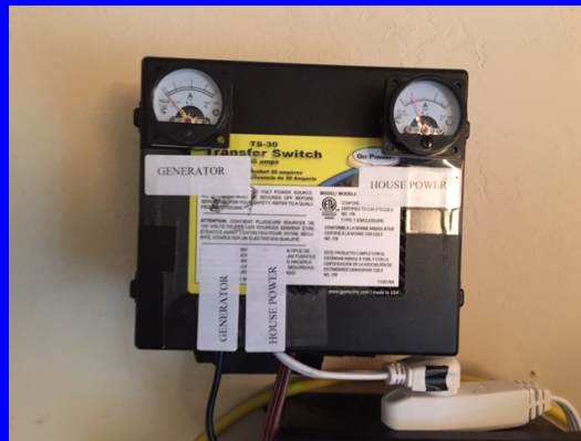
House to Gen Transfer Switch
