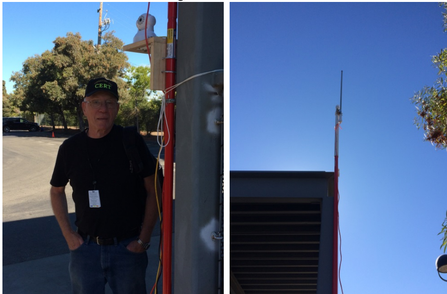
Doug standing by the mast strapped to an enclosure with the webcam mounted just above his head. A power supply box (not shown) also holds the POE injector for the Ubiquiti as well as the 12vdc to 5vdc adaptor for the camera.
