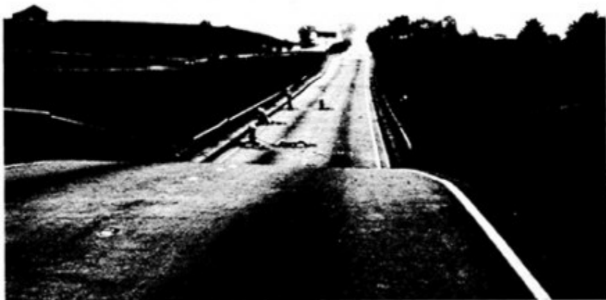
FIGURE 6-5 Collapsed Struve Slough Bridge.
