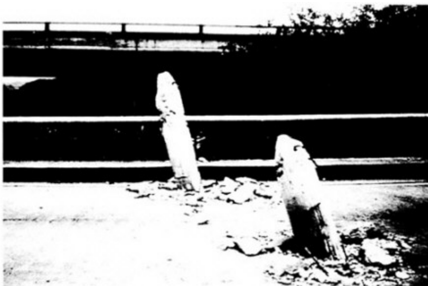
FIGURE 6-8 Piling penetrated six-inch deck between girder stems.
